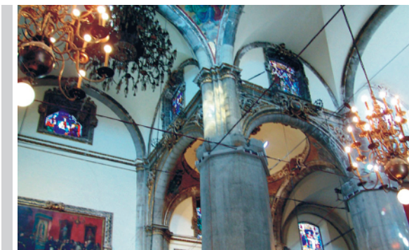
Figure 9. Steel ties-temporary protections of pillars [35]
