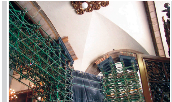
Figure 8. Temporary protection of arch [35]
