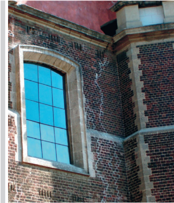
Figure 6. Trace of repair of facade masonry of „old” Basilica [35]
