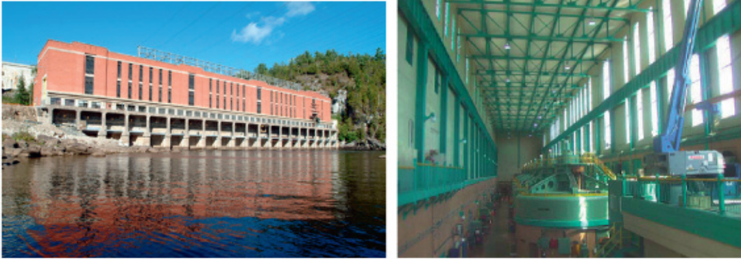
Figure 4. The outside and inside views of the powerhouse
