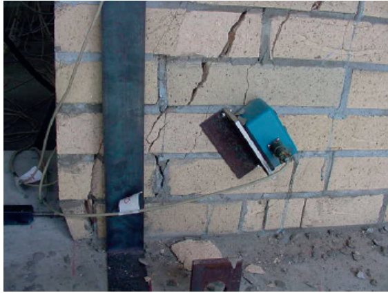
Figure 8. Side and end views of toe crushing in reinforced grouted
