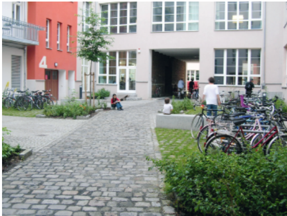
Figure 14. An example of rebuilding of the western part of Berlin: The new image of old inner gardens in-between living houses. Photo: The author
