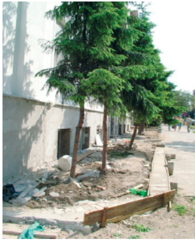
Figure 4. Earthworks within the root system. There has been a disclosure and damage of the roots and soil chemistry change as a result of long-term retention of alkaline soil materials, Kochanowskiego Street, Poznan. [Own photograph]
