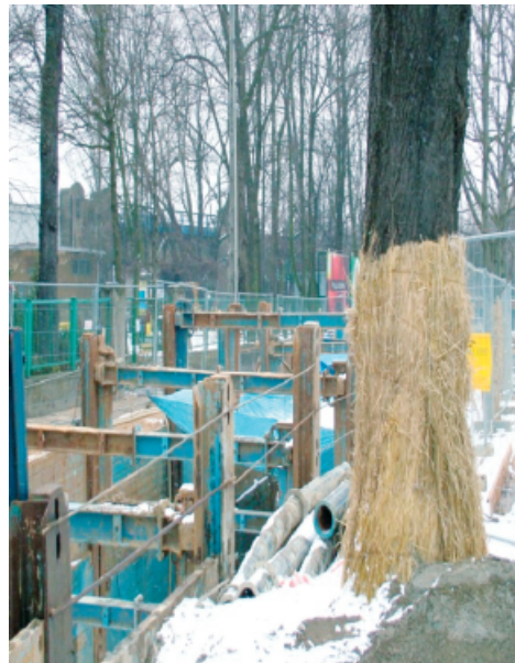
Figure 2. Construction of collector sewers, Poznań [Own photograph]
