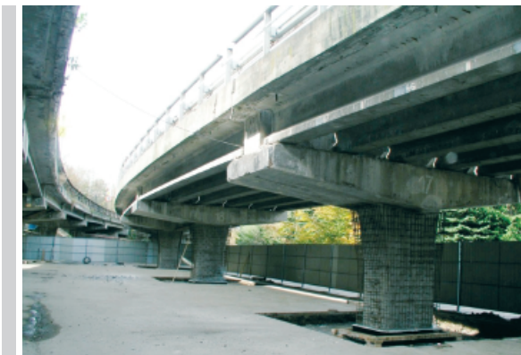
Figure 1. View of viaduct before repair
