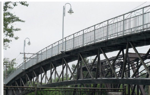
Figure 1. General view of Sherbrooke footbridge (left-hand side)
